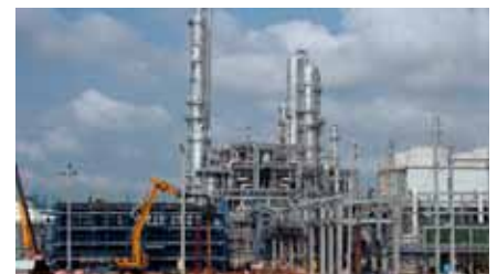
Propylene Glycol Project
