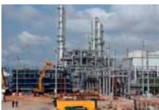
Propylene Glycol Project
