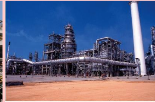
Thaioil Hydrocracker (HCU)-2 538 THBmn, Chiyoda
