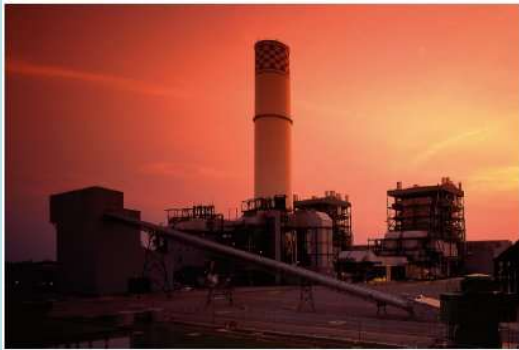
Ratchaburi Power Plant 4,394 THBmn, RATCH
