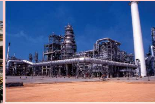
Thaioil Hydrocracker (HCU)-2 538 THBmn, Chiyoda
