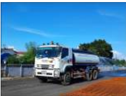
Photo depicting water spraying to reduce dust dispersion, speed limit for vehicles, and cleaning of wheels before leaving the construction site.
