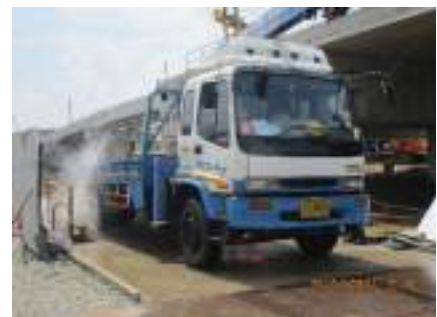
Photo depicting water spraying to reduce dust dispersion, speed limit for vehicles, and cleaning of wheels before leaving the construction site.
