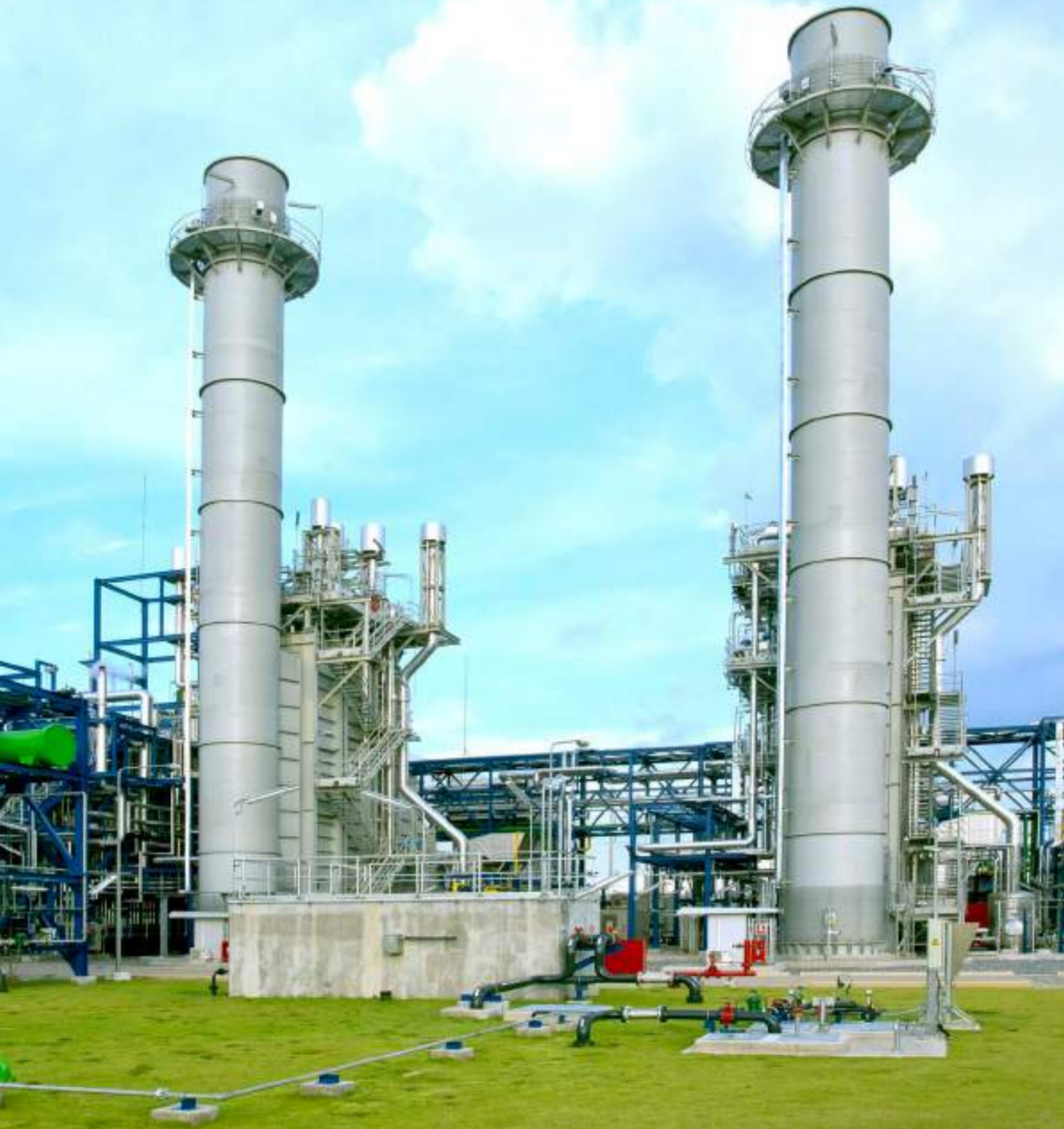
Ban Lane Power Plant, Ayutthaya
