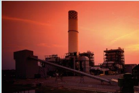
Ratchaburi Power Plant 4,394 THBmn, RATCH
