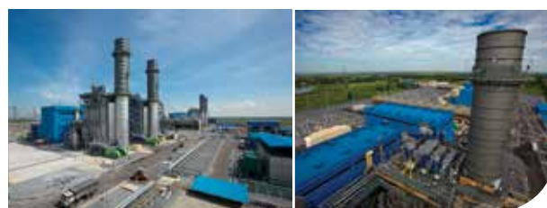
GJP-GNS and GUT combined Cycle Power Plants
