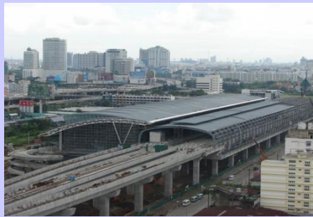
Airport Rail Link 13,225 THBmn, SRT
