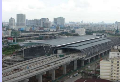
Airport Rail Link 13,225 THBmn, SRT
