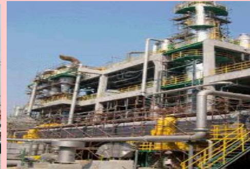
Thai Olefins Plant Expansion 1,262 THBmn, TOC
